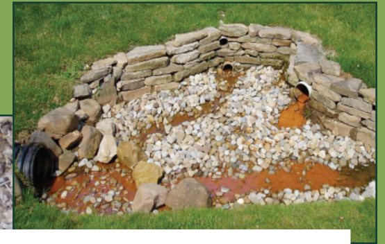
Iron, algal growth, and resulting oil-like sheen
